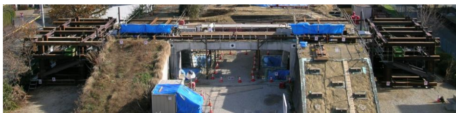
Figure 3. A general view of the model with arrangements for lateral loading tests (Koda et al., 2013).
